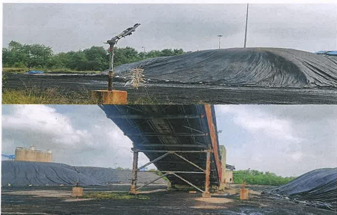
**Dust extraction system at coal handling area**
